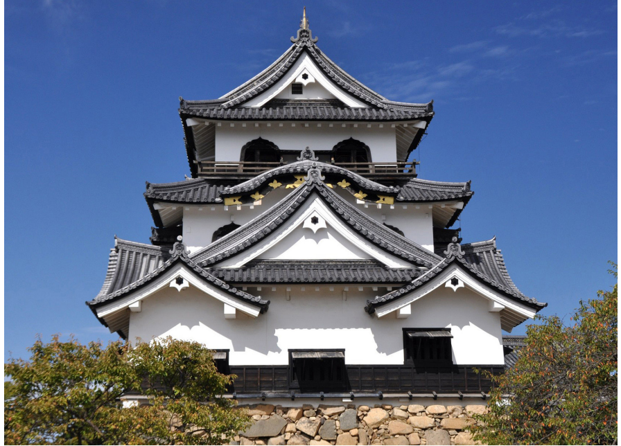
Hikone Castle's tower was moved and rebuilt from other castle which tower castle was four layers and five floors. Is has a history unique to wooden architecture which is easy to dismantle, transport, and rebuild. 1-1 Konkicho, Hikone-shi, Shiga http://www.hikoneshi.com/jp/castle/
